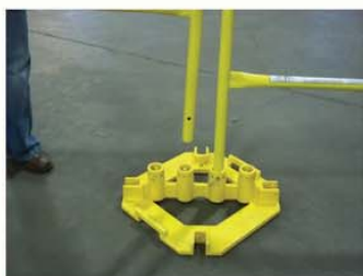
Set base in place and insert railing section.
